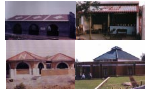
Fine examples of Micro-Concrete Roofs
