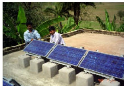
Figure 6. Installing PV modules on the village clinic
